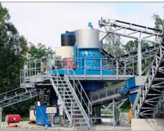
Cone crusher KDC 35 FP - greywacke crushing
