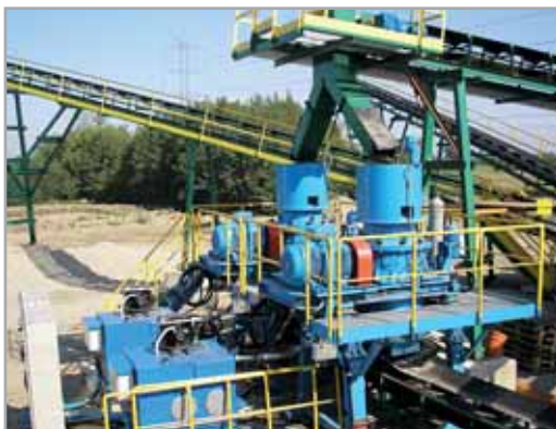
Tertiary crushing with crushers KDC 32 JP
