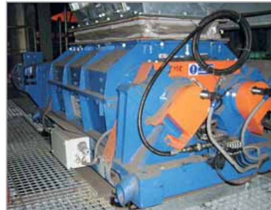
Crusher DVR 18 – slag crushing 12t/h
