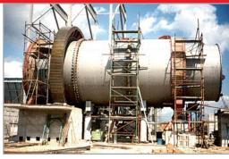
Assembly of a raw mill Ø 5.4 x 11 m with pre-drying chamber
