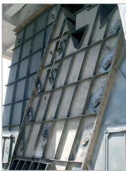
View of the separator upper part with the material inlet and gas exhaust
