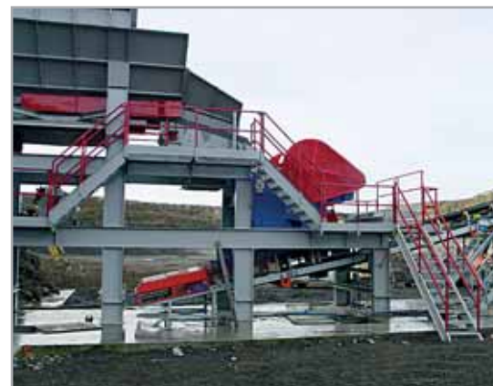
Jaw crusher DCJ 1039 - basalt crushing
