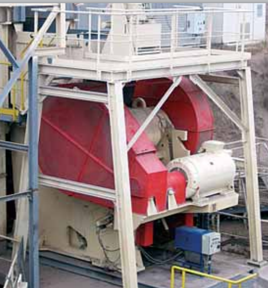
Jaw crusher DCJ 1038 – basalt crushing
