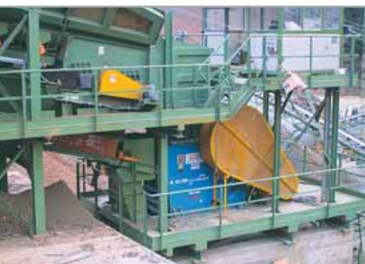
Jaw crusher DCJ 1021 – basalt crushing
