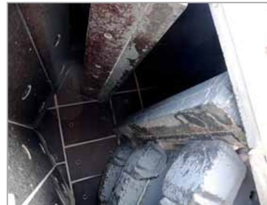
Crushing area of the crusher ODH 1110-23
