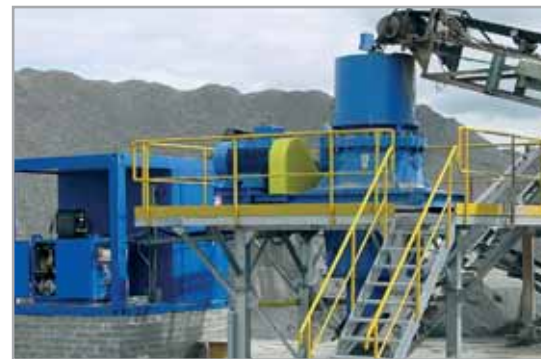
Cone crusher KDC 33 JP – spilite crushing
