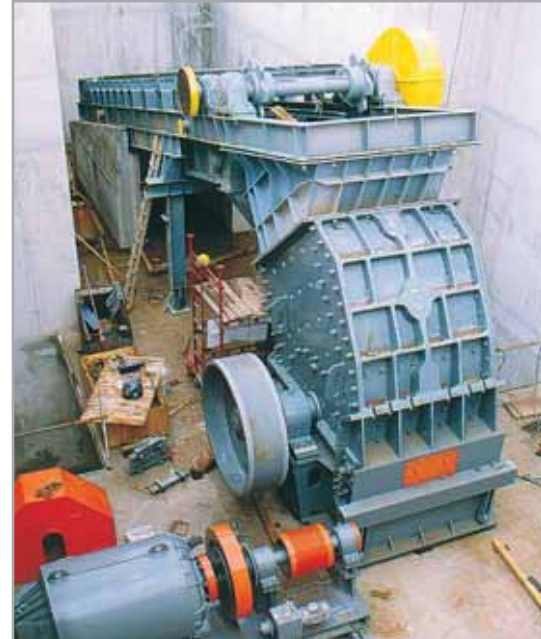
Assembly of the apron feeder CPLDT 1600x12000
