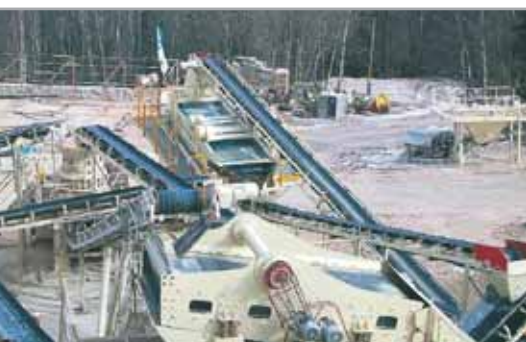
Vibrating screen EDN-2N 2050/2 – felspar screening
