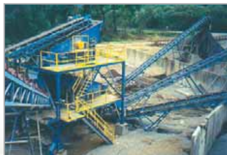
Vibrating screen KDT 2050/2 – andesite screening
